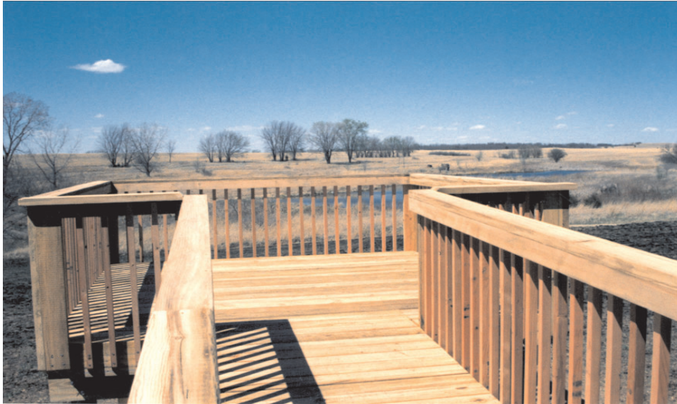
Lumber milled from utility poles is donated for local projects, such as this wildlife-viewing platform. Photo by Brad Loveless
